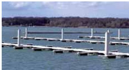
Abb. 13: Anlage in Chantecog
